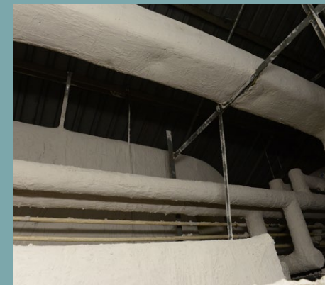
冷水管及風管 (施工後) Chiller water pipe and air duct (After application)
